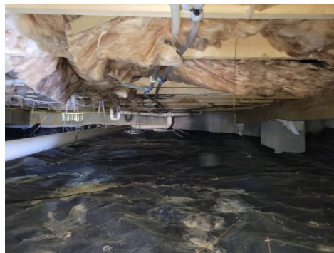
View of crawlspace.
