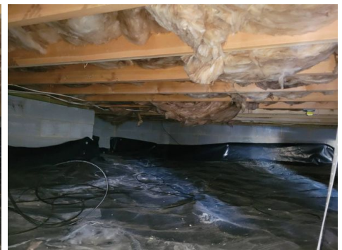
View of crawlspace.
