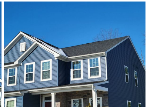
View of roof.
