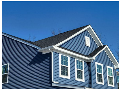
View of roof.
