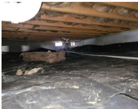
View of crawlspace.
