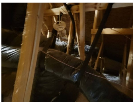
View of attic.
