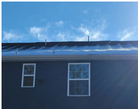
View of roof.
